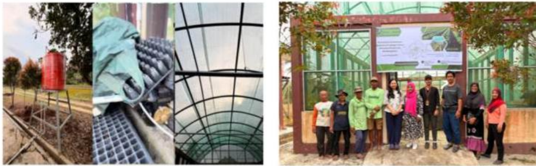
Figure 5 Installation of key greenhouse infrastructure and community training session with local farmers at TTP
